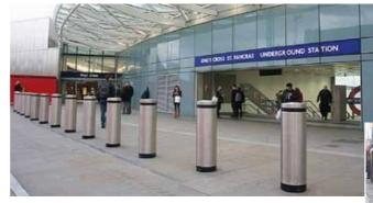
Kings Cross Station, London - bollards designed to withstand vehicle impact
