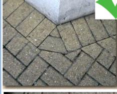
Paving laying should be orientated to follow the grain when using paving chamber covers.
