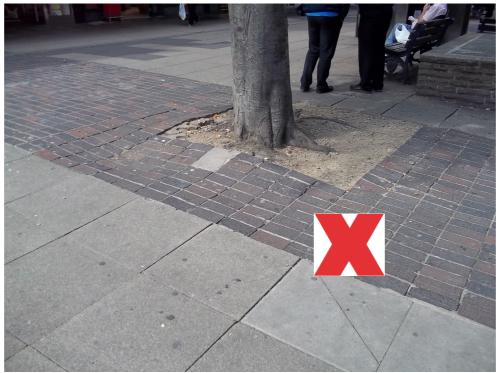
Rigid paving construction ensures the longevity and durability of the finished surface, unlike flexible paving systems which sink, move and distort. Street reinstatement works should be carried out in accordance with: <a href="https://www.gov.uk/government/uploads/system/uploads/attachment\_data/file/4382/practicalguidetostreetworks.pdf">https://www.gov.uk/government/uploads/system/uploads/attachment\_data/file/4382/practicalguidetostreetworks.pdf</a>
