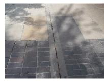
Drainage should be carefully considered, slot drains are aesthetically pleasing within a scheme, but the width of the gap should be considered to avoid trapping debris and cigarette butts, which inhibit the drains function.
