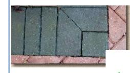
Paving laying methods should be considered carefully at junctions to achieve a larger fill piece. As shown in the two examples to the
