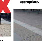
Stud tactile pavers or brass studs are required at pedestrian crossings and corduroy at level changes. These should be designed sensitively and sensibly. Studs should be raised enough to serve their purpose but not overtly proud. Where possible tactile units should be made of matching materials to the surroundings.
