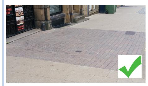
Vehicle dropped crossing details to be made up in small Tegula sett details which allow them to follow the contours of the ground better. This gives a better result
